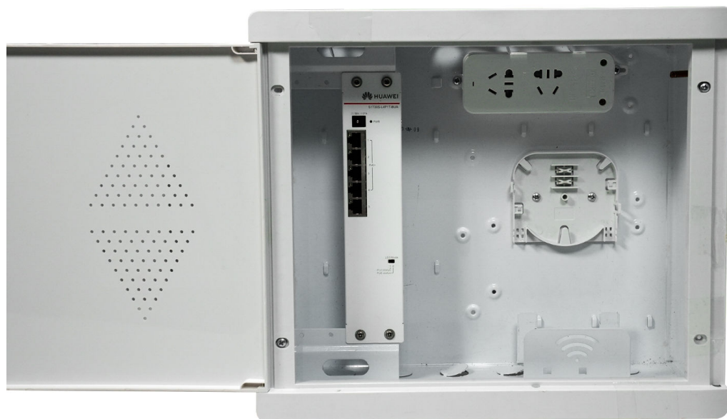
Figure 3-28 Installing a switch in a network box
